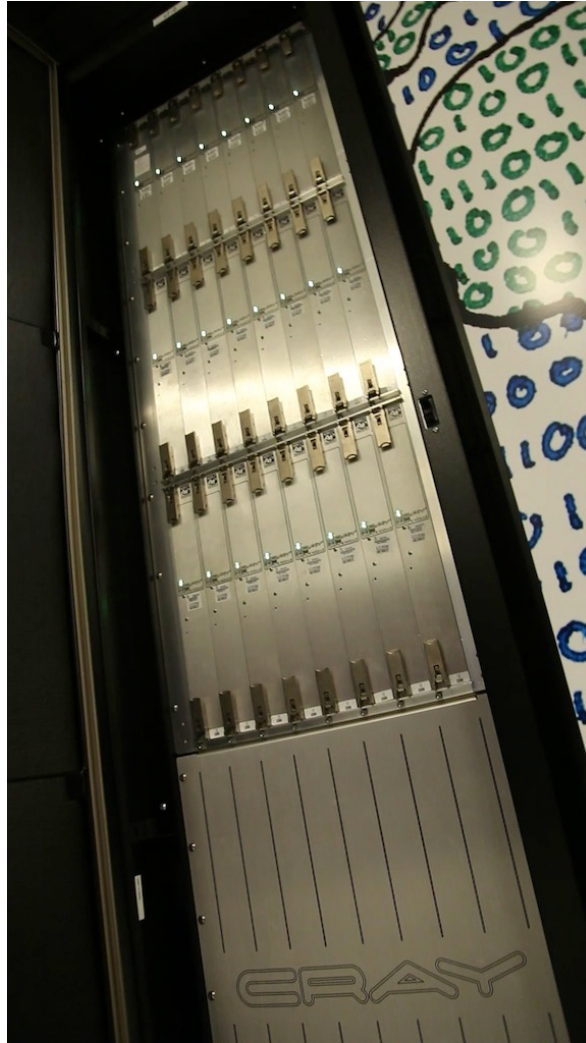
Figure 4: Inside One of HECToR's Cabinets [4]
